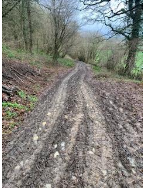
Figure 3: Waterlogged path after significant rain
