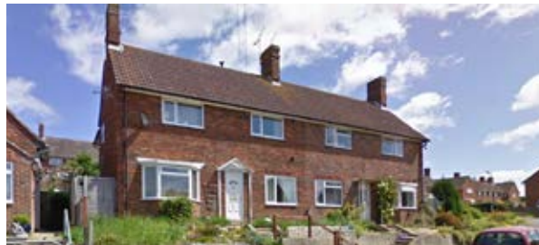
Topography rising at Blackdown with landscaping retaining a positive relationship with the street
