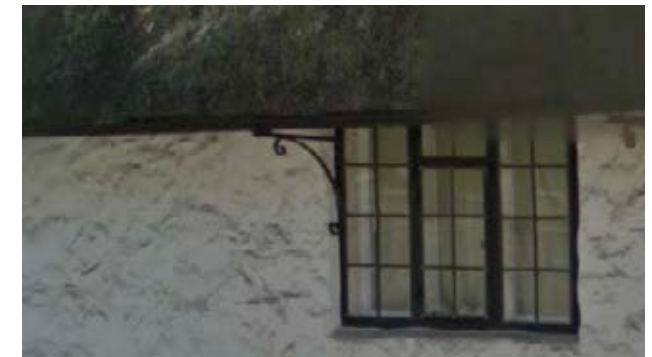
Painted Cobb and thatch roof
