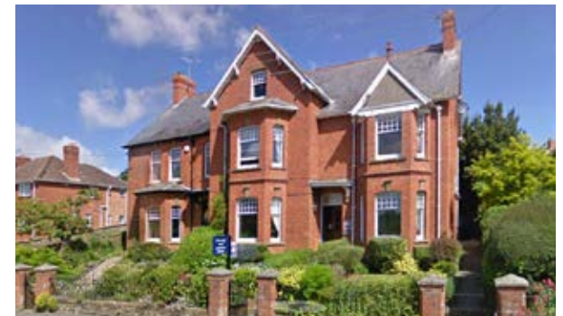
Villa set above the street with a positive relationship of surveying the street but maintaining privacy.
