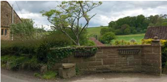
Boundary wall is low to offer views out to the rolling hills and natural environment.
