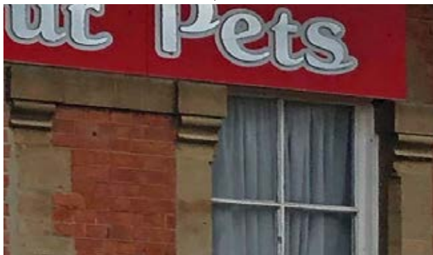
Brick built building with stone detailing to the corners and sash windows
