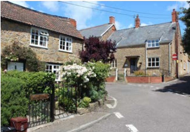
Traditional 2 storey cottages with gable ends and attractive relationships with the street. Roof changes to remove bulk of semi-detached with the rise in the road.
