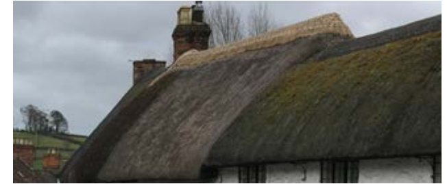
Thatched roofs with brick chimneys.
