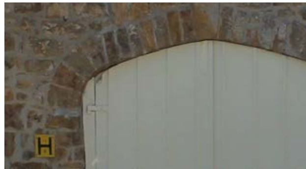
Traditional stone detailing to the garage door
