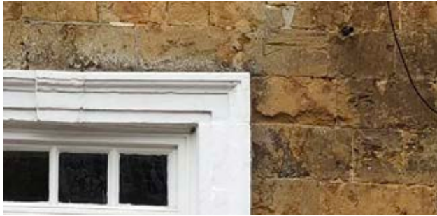
Wooden door surrounds and traditional stone details and Georgian window divides.
