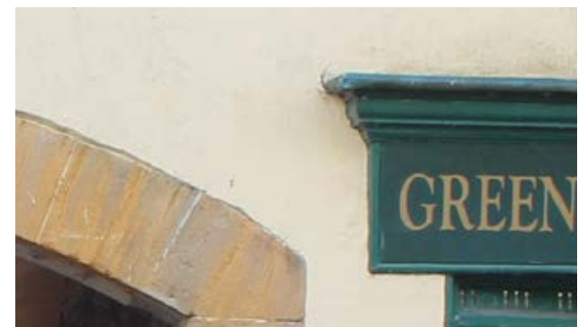
Painted wooden shop front with painted render to the walls and stone detailing.
