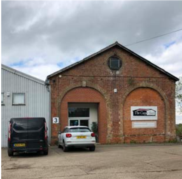
Typical industrial building
