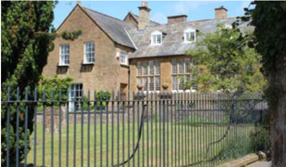
Typical dwelling in Historic centre constructed of stone with a slate roof
