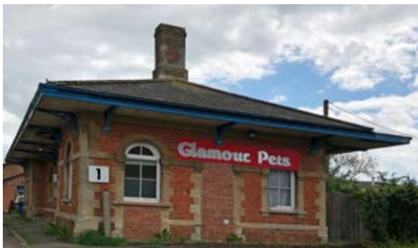
Industrial building with contrasting lintels
