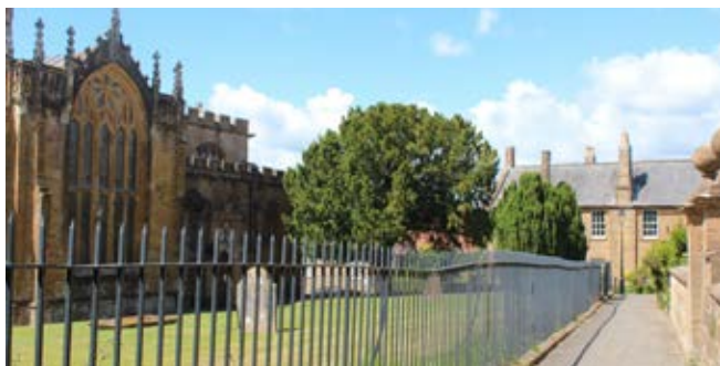
The low wall defines a clear boundary whilst offering views to the Minster and green space behind.
