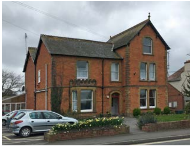
Large detached Victorian Villa with potential to be converted into multiple units but appear as a single unit
