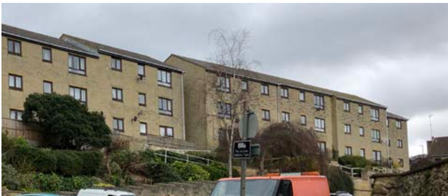
Utilitarian and placeless design with blank façades and no roof detailing. An imposing scale out of keeping with the topography.
