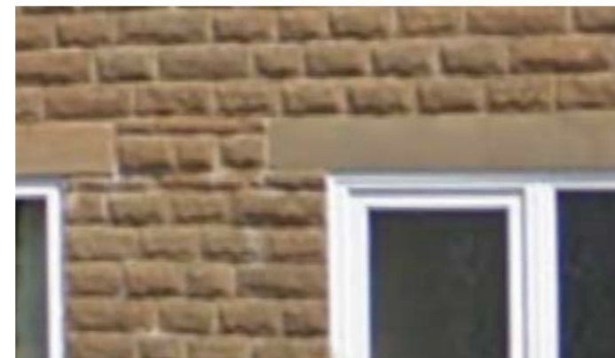
Faux stone with no or plain window details that are poor quality, foreign to the area and out of keeping with the local context.
