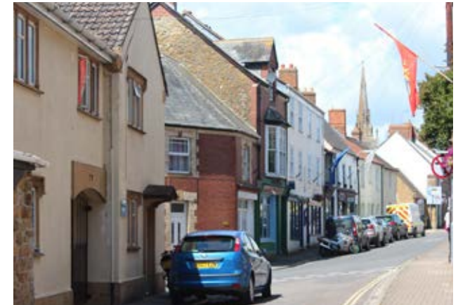
Mixed property types, up to 3 storeys in height with varying widths and shapes that create interest.
