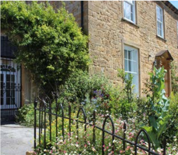
Attractive small private front gardens to store bins with attractive stone walls and metal railings
