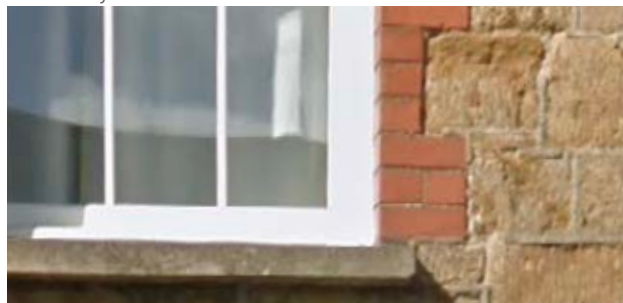
Traditional natural stone building with brick detailing, stone sill and sash windows
