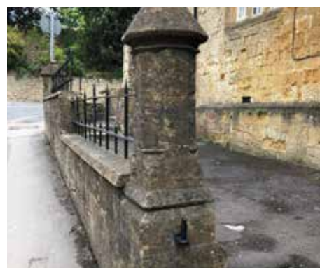
6. The staggered boundary wall, reducing in height close to the entrance point, visually aids way-finding.
