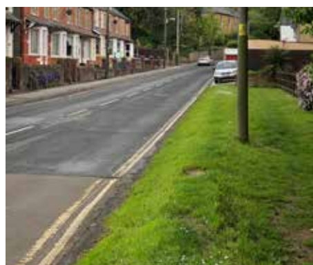
8. Pathways to both side of the road are not provided again reflecting the towns rural heritage.
