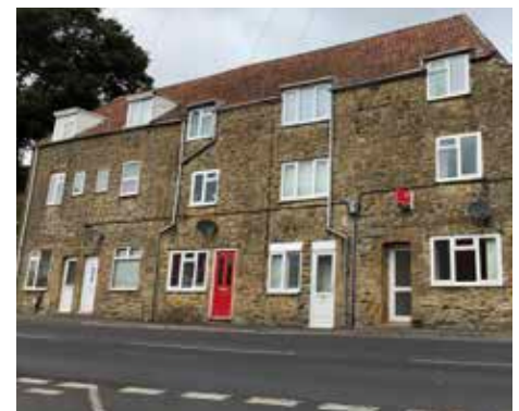
9. Moolham stone façades are also a characteristic of the area, nicely blending with the Hamstone's warming tone.
