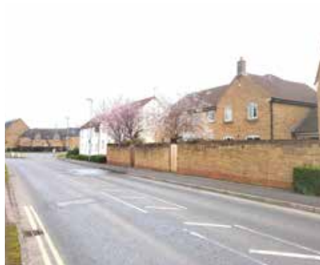
13. This traditionally rural style boundary treatment reflects the urban/rural edged nature of this development.
