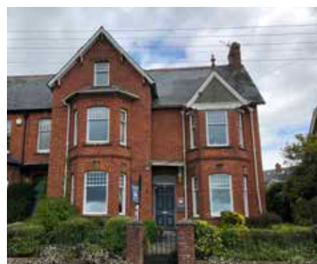
9. Brick pillars offer grandeur to the entrance, with soft, low boundary treatment nestling the building.
