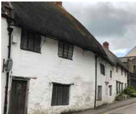
4. Medieval buildings with ad-hoc fenestration.
