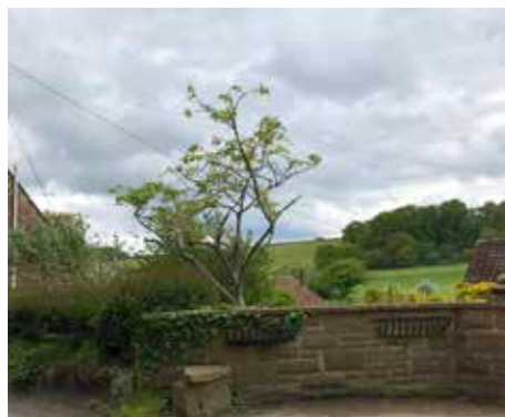
1. Boundary wall is low to offer views out to the rolling hills and natural environment.
