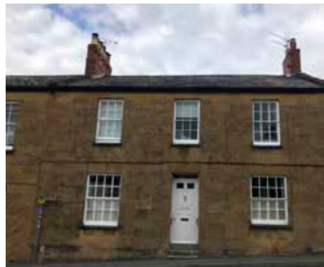
3. Fenestration is simple and elegant, reflecting architectural heritage and cottage-style proportions.
