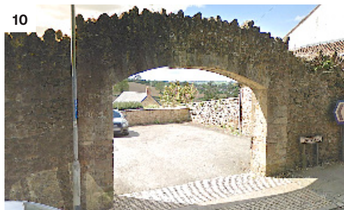
10 Townsend View from north-east Townsend Road to Pretwood Hill to the south.
