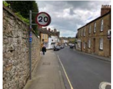
3. Pathways are narrow emulating countryside tracks, as a result these cause accessibility issues in some areas.
