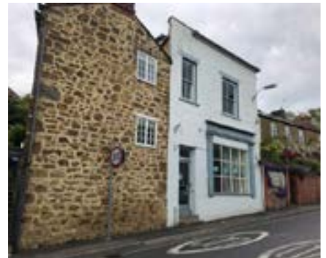
3. Where properties break from using Hamstone a similar tone is used with brick Moolham stone or paint.
