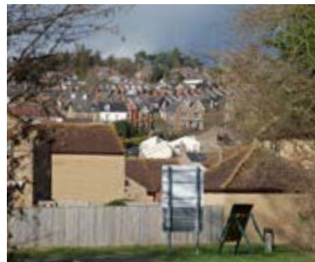
15. The southern green ridge and development on the northern ridge are very visible within Ilminster.
