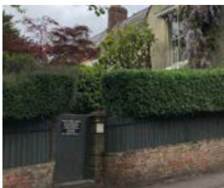
5. Mix of boundary wall materials unique to building offer privacy and a soft appearance, greening the street scene.
