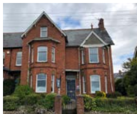
9. Brick pillars offer grandeur to the entrance, with soft, low boundary treatment nestling the building.
