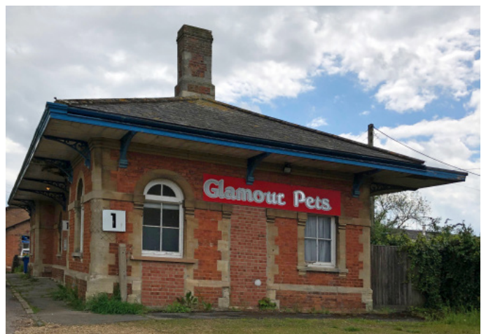
Industrial building with contrasting lintels
