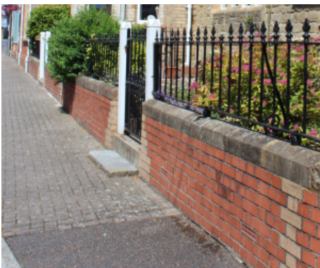
Decorative railings offer a distinct separation between private and public space on narrow pathways.
