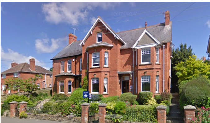
Villa set above the street with a positive relationship of surveying the street but maintaining privacy.
