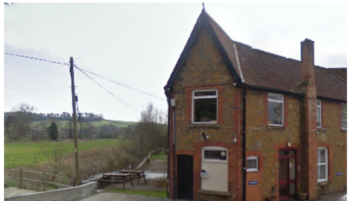
Far-reaching views beyond Rose Mill industrial estate.
