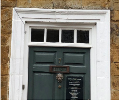
Wooden door surrounds and traditional stone details and Georgian window divides.
