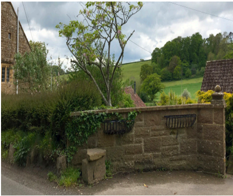
Boundary wall is low to offer views out to the rolling hills and natural environment.
