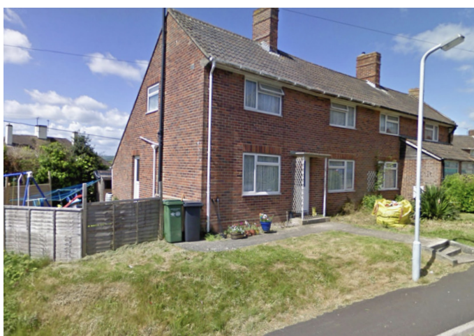
Typical gable end and red brick with chimneys
