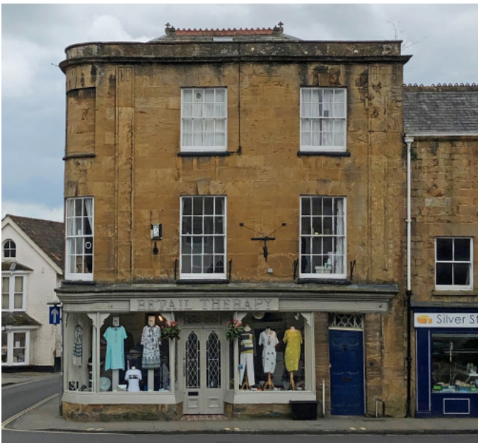
Typical historic centre building
