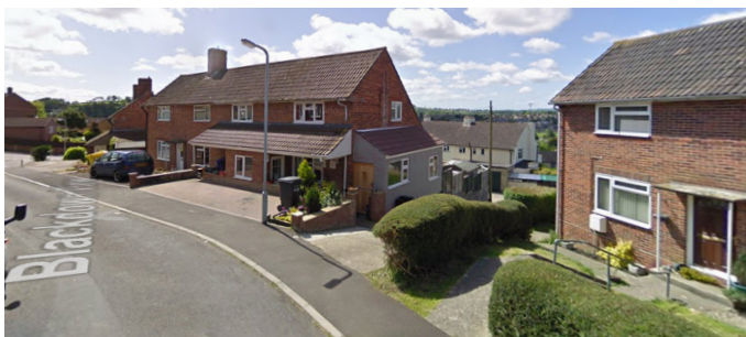
Topography falling at Blackdown View retaining a positive relationship with the street and privacy without boundary treatment needed.
