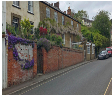
A mix of boundary wall and materiality of the buildings promote an appearance that is unique to every house.
