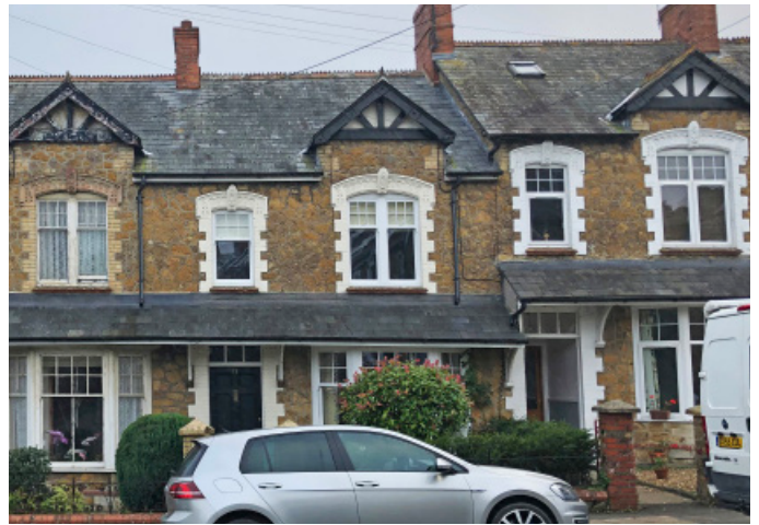
Typical terrace with ornate window details
