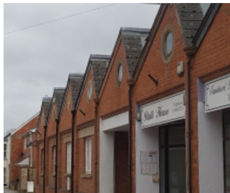
Industrial gable ended roof forms creating interest.
