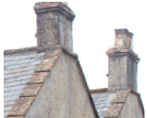
Rendered gable ends, coping stones and rendered chimneys.
