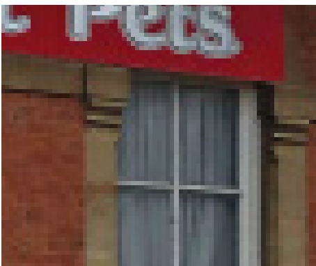
Brick built building with stone detailing to the corners and sash windows.
