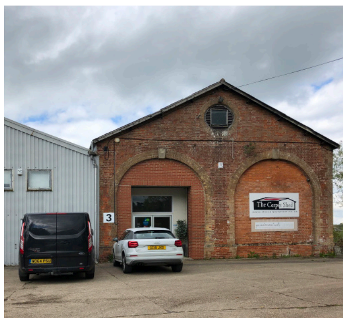
Typical industrial building
