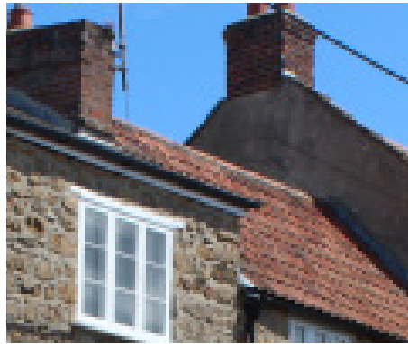
Clay tile roof with brick chimney, hipped away from the street but at varying heights within the terrace.
