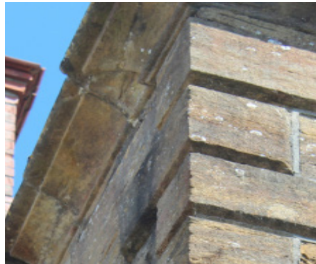
Stone detailing to the corners and soffit with a brick chimney.
