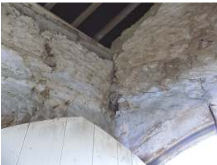
Walls to covered area
