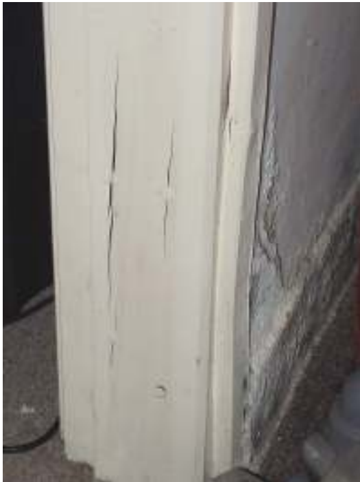
Internal door frame to main bedroom
