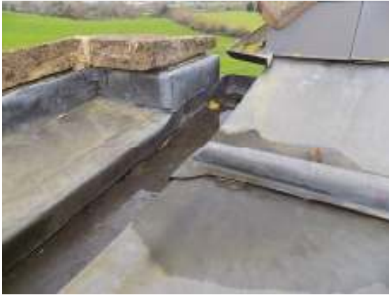
Water to lead gully
