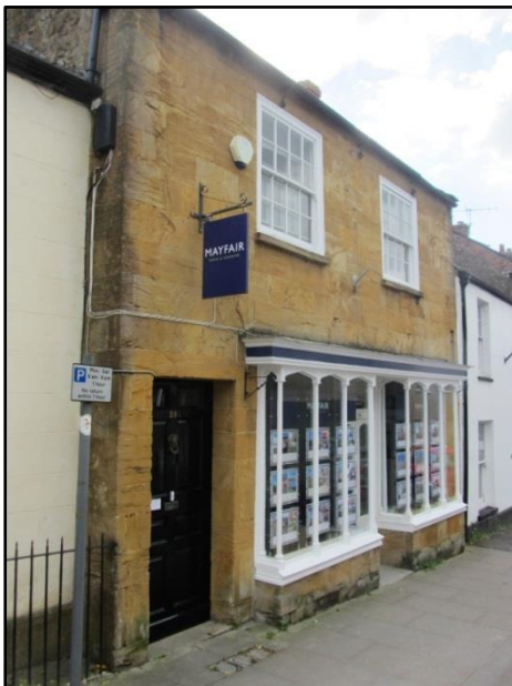
Shopfront in East St
